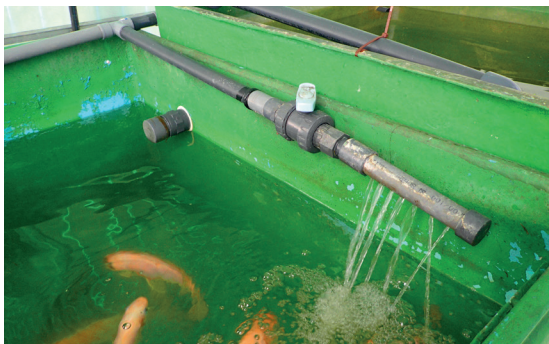
Retorno de agua al recipiente / Water return to the tanks
